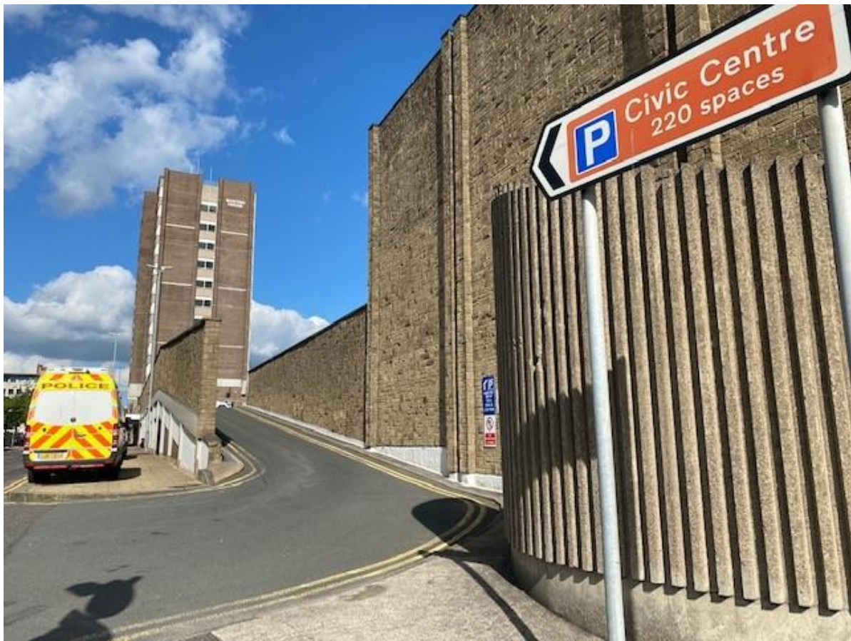
Buxton House and the car park ramp from Albion Street looking North
