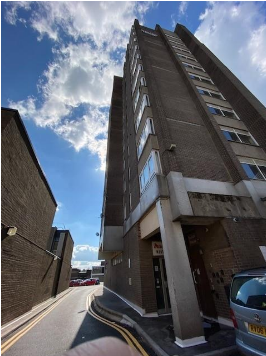
Buxton House looking South with access roadway to the East
