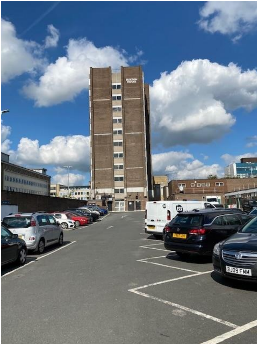
Buxton House and first floor car park looking North
